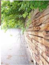
You may have noticed the old wooden retaining wall mostly out from the 55 building. It is bulging badly and is destined for collapse someday. Rather than wait for that to happen, work will start shortly on a new classy boulder wall. Boulder walls are incredibly strong and, although, a bit more expensive than Keystone walls, look hope to get vegetation to grow right amongst the boulders.
